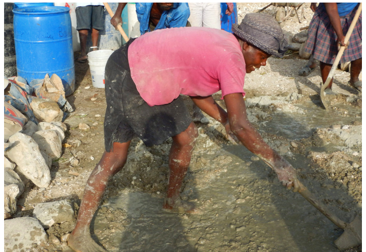
Photo: A woman mixes concrete for the school's new foundation.
