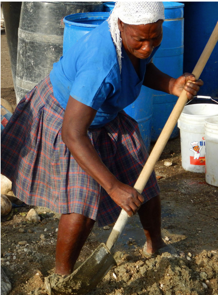
Photo: Despite issues of severe gender discrimination found throughout Haiti, men and women are equal on the buildOn worksite.
