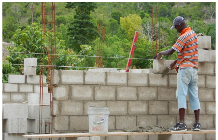
Photo: It take over 3,000 bricks to construct one buildOn school.
